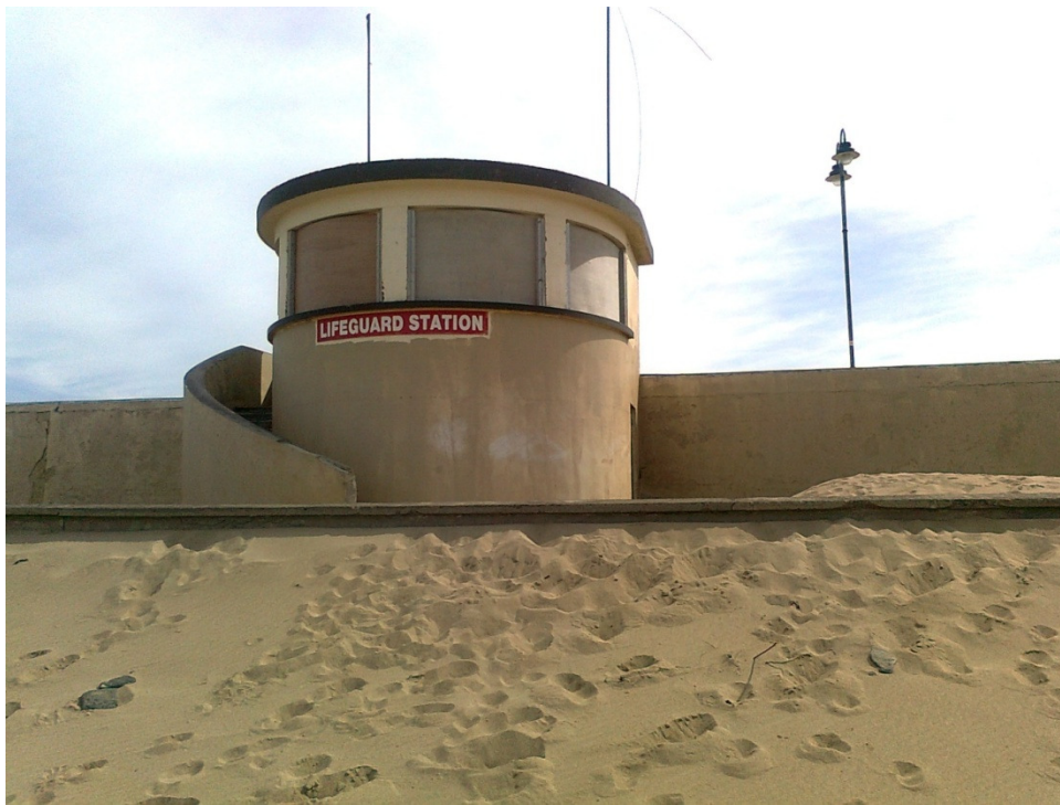
Plate 1. Bundoran Lifeguard Station before facelift.
